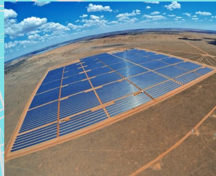
50MW Droogfontein Solar PV
